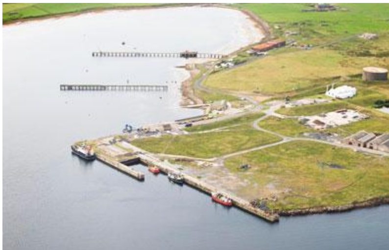
Port of Lyness before development. Source: Orkney Island Council Marine Services (2011a) Marine Renewable Energy Strategy
