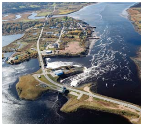
The Annapolis Royal Generating Station.
