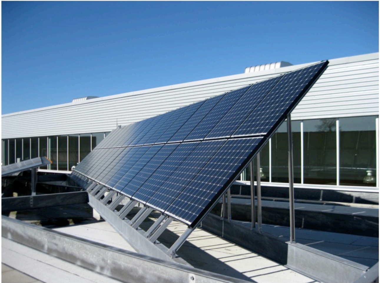
Solar photovoltaic array at Nova Scotia Community College, Dartmouth, NS Photo: Wayne Groszko
