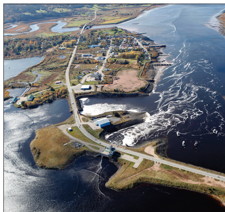
Annapolis tidal barrage installed in 1984. The plant generates up to 20 megawatts, enough power for up to 6,000 homes.
