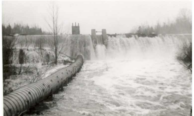
Picture 1 Hydroelectric Dam and Penstock, Factorydale, NS Courtesy of Berwick Electric Commission
