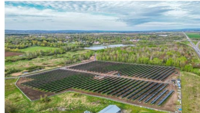
Image 1 Berwick Community Solar Project. Photo Credit - Communications Nova Scotia
