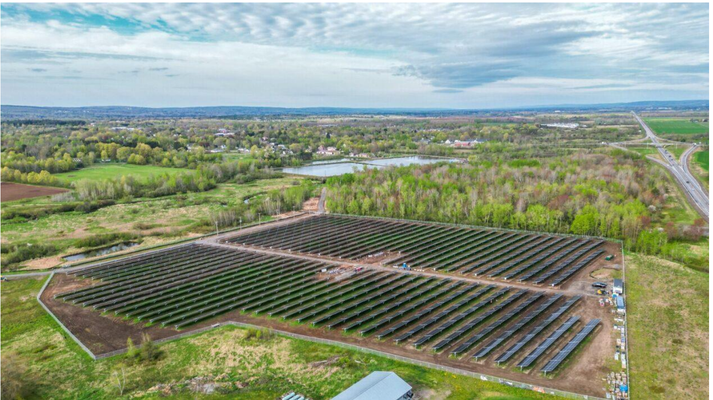
Image 1 Berwick Community Solar Project. Photo Credit - Communications Nova Scotia
